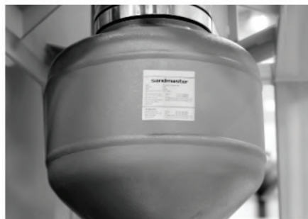
Pressure vessel installation
